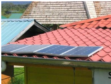
Fig.5 Solar panel installation on Bario TeleCenter's rooftop.
